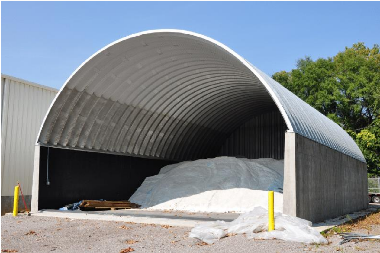
Road Salt Storage
